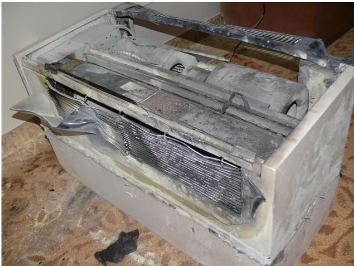
Failure of compressor leads on hotel HVAC unit
