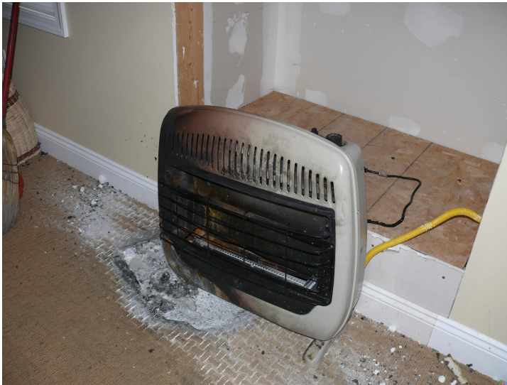
Failure of gas heater installation
